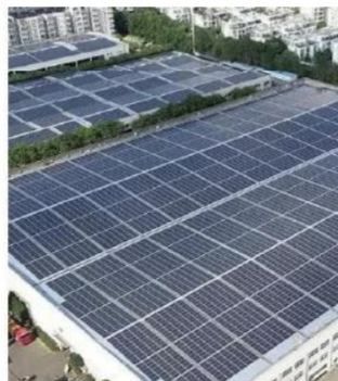
Industrial and Commercial Roof
