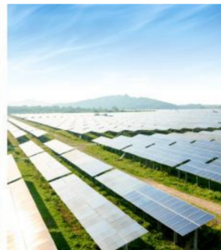
Array Power Station
